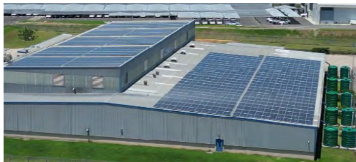
We focus on conserving resources and using renewable energies: in 2023, we commissioned our solar plant at our site in South Africa. This will enable us to cover up to 12% of our electricity requirements. We also use collected rainwater for cooling, thereby reducing fresh water consumption.
